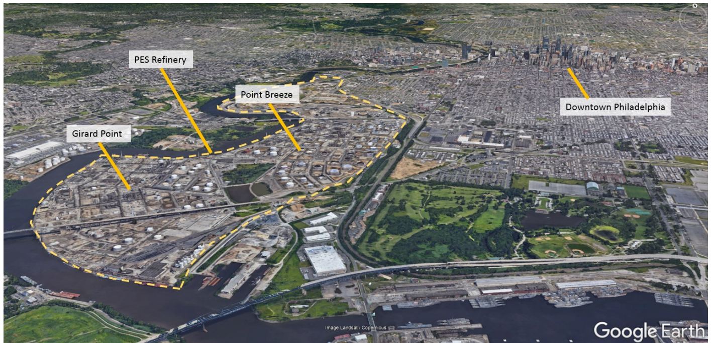
Figure 1. Overhead view of the PES Refinery in Philadelphia, Pennsylvania, showing the Girard Point and Point Breeze refineries. (Credit: Google Earth with modifications by CSB).
